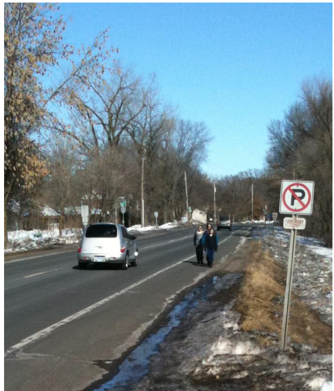
TH 96 today (before resurfacing)
