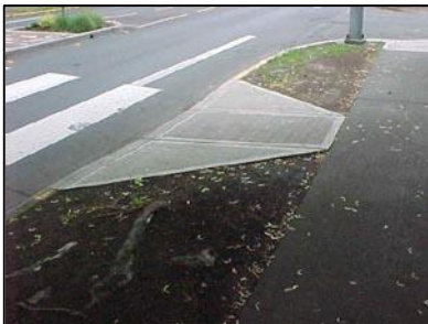
Pedestrian Curb Cut/ADA Ramp Source: City of Portland
