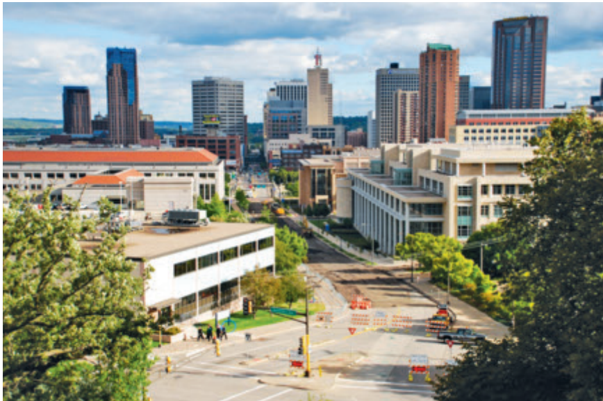
St. Paul: Robert Street's surface is removed between University Avenue and 12th Street, the first day of construction, September 7, 2010, on the Central Corridor LRT.
