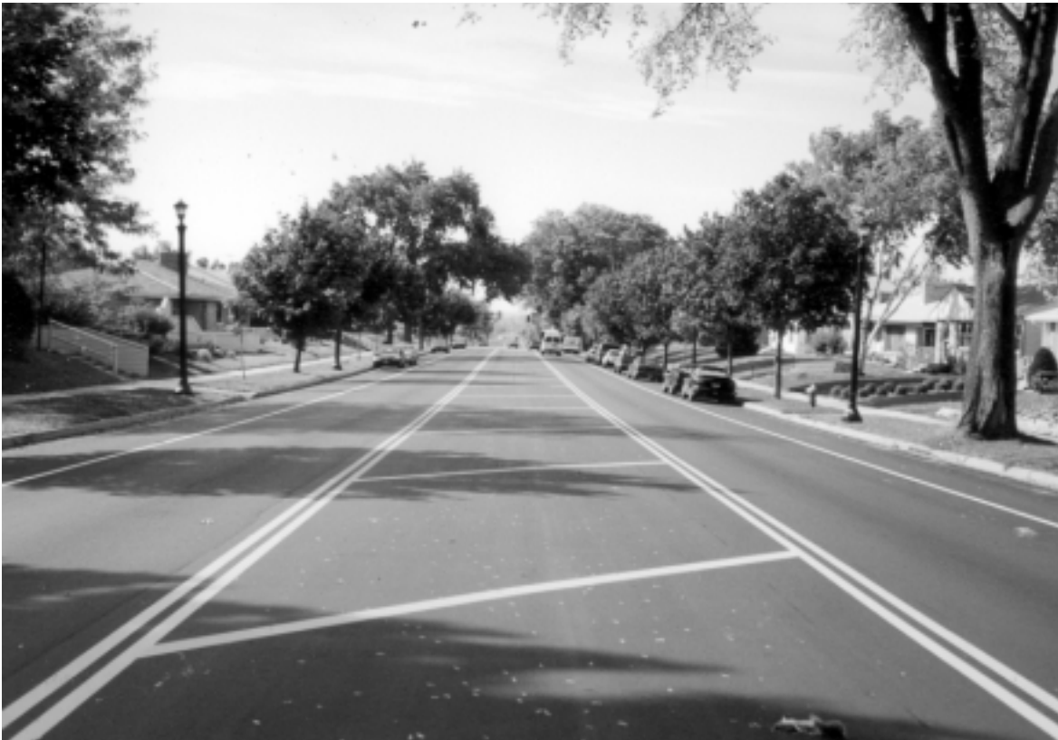
Ford Parkway in Saint Paul. Saint Paul has converted a number of roads from four lanes to two with a center left-turn lane, and accident rates and speeding have declined. This design is encouraged by MnDOT.
