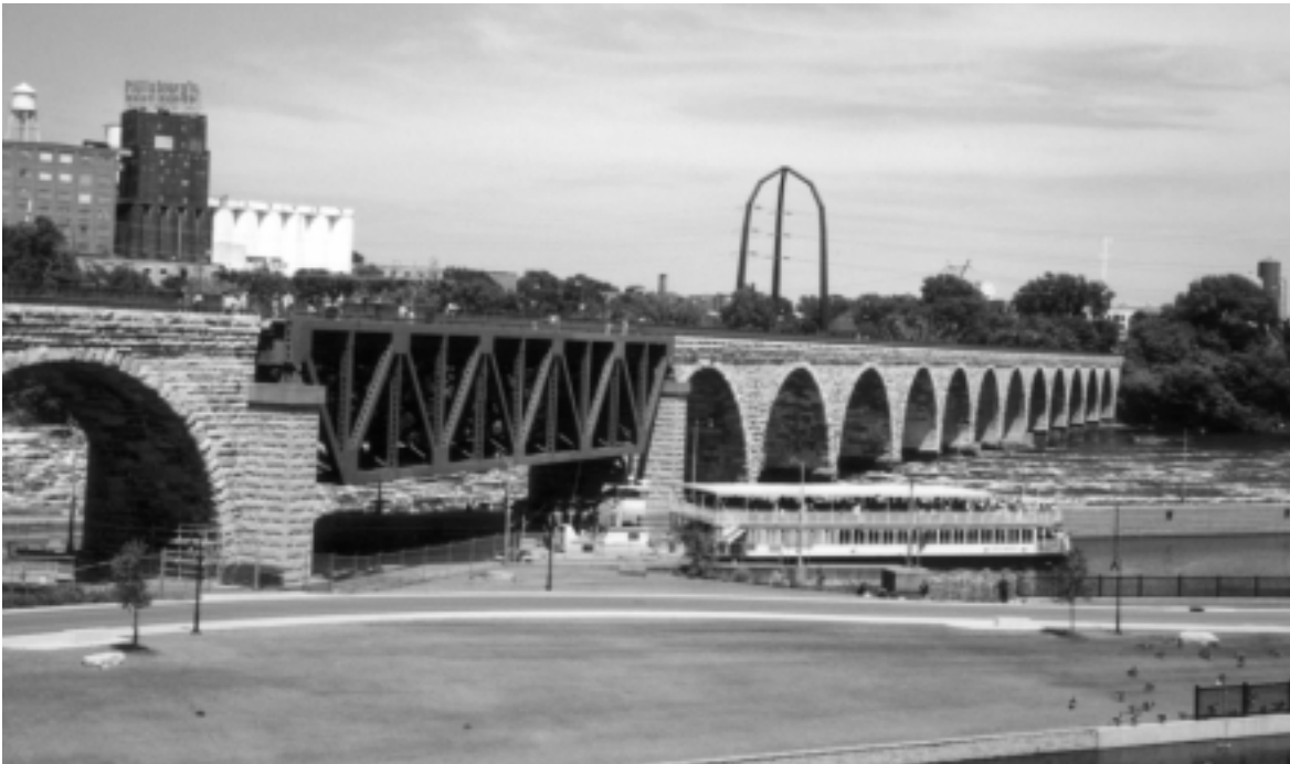
Federal transportation funding is often used for major bike and pedestrian projects such as the Stone Arch Bridge in Minneapolis.
